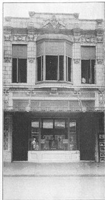
Office and Retail Store.
